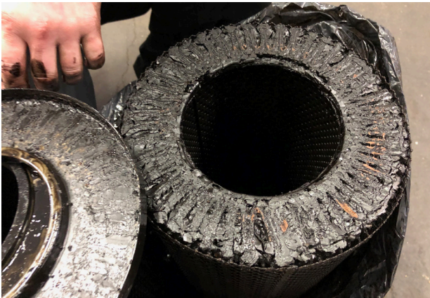
A result of non-optimised fuel blending
